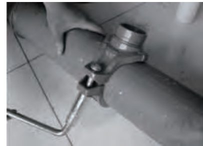
6. Secure the nuts and bolts of side outlet from both side.
